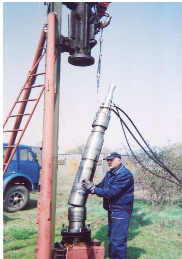
Fig. 5. Mounting of IRE propelled diesel pile fixing hammer.
