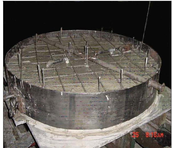
Fig. 2. Reinforcement rodings placed inside the metal box.
